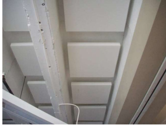
Figure 2: Concrete deck AFTER
