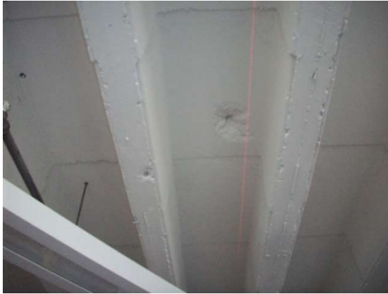
Figure 1: Concrete deck BEFORE
