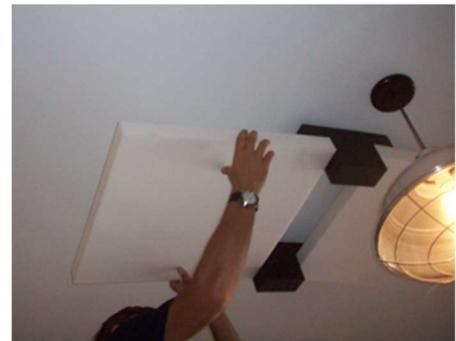
**Positive Fastening:** Where substrate is subject to thermal change, such as metal roof decks, use a positive fastening system. Attach standoffs to flutes of deck with self-tapping screws and large washers. Adhere panels to standoffs; putty knife application is recommended.
